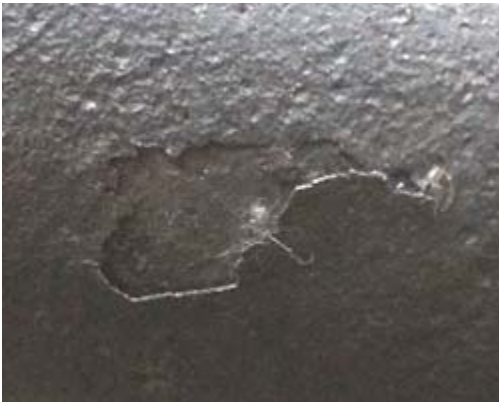
Stripping defect
