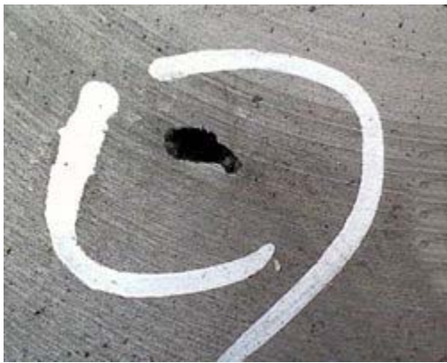
sand hole defect
